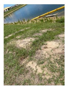
**Location 4:** Bare soil observed. Lack of vegetation/sod makes the bank prone to erosion. Sod all disturbed areas.
