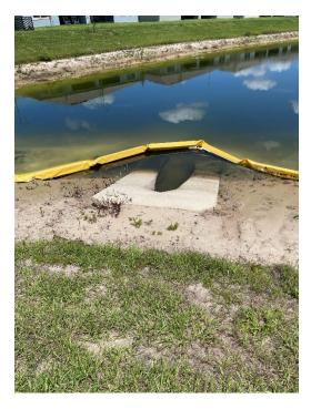
**Location 13:** Bare soil observed around the control structure. Lack of vegetation/sod makes the bank prone to erosion. Sod all disturbed areas.
