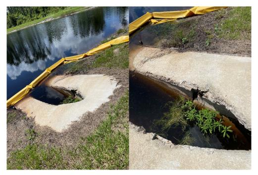
**Location 2:** Bare soil observed. Lack of vegetation/sod makes the bank prone to erosion. Sod all disturbed areas.
