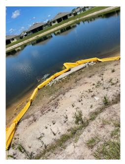
**Location 14:** Bare soil observed around the control structure. Lack of vegetation/sod makes the bank prone to erosion. Sod all disturbed areas.
