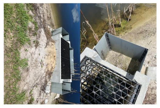
**Location 12:** Turbidity barrier was installed and not removed. If construction is completed the turbidity barrier should be removed. Evidence that the mitered end section (MES) is starting to get undermined.
