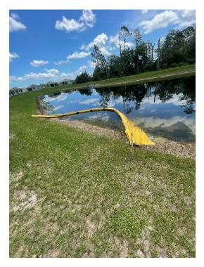
**Location 11:** Bare soil observed around the control structure. Lack of vegetation/sod makes the bank prone to erosion. Sod all disturbed areas.
