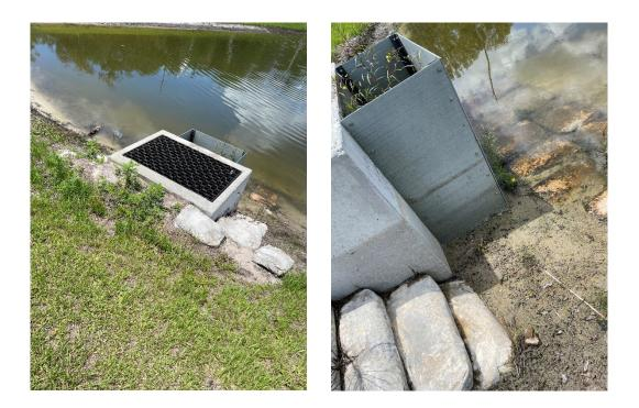
**Location 16:** Existing trees are to be removed that are crossing the sump area. Ditch pavement is starting to show signs of erosion and undermining. We recommend rip rap around the existing outfall structure to deter undermining and erosion.
