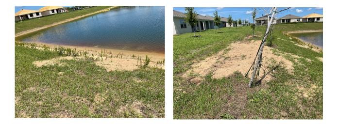
**Location 5:** Bare soil observed. Lack of vegetation/sod makes the bank prone to erosion. Sod all disturbed areas.
