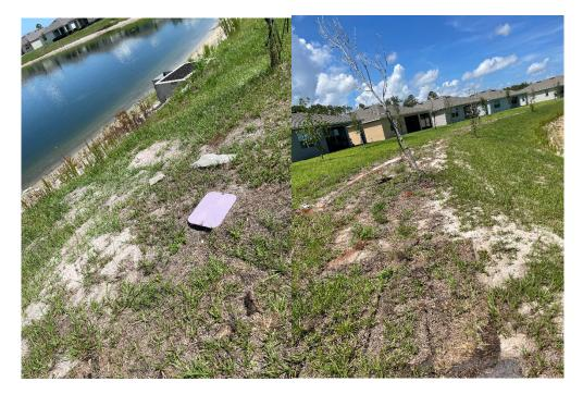
**Location 3:** Bare soil observed. Lack of vegetation/sod makes the bank prone to erosion. Sod all disturbed areas.
