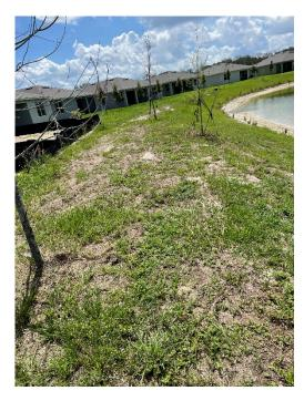
Location 9: Exposed bond bank is prone to erosion. Sod exposed pond bank to prevent future erosion
