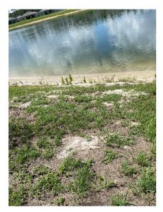
**Location 8:** Bare soil observed. Lack of vegetation/sod makes the bank prone to erosion. Sod all disturbed areas.
