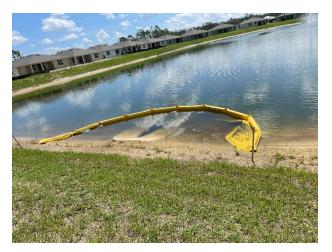
**Location 7:** Bare soil observed. Lack of vegetation/sod makes the bank prone to erosion. Sod all disturbed areas.
